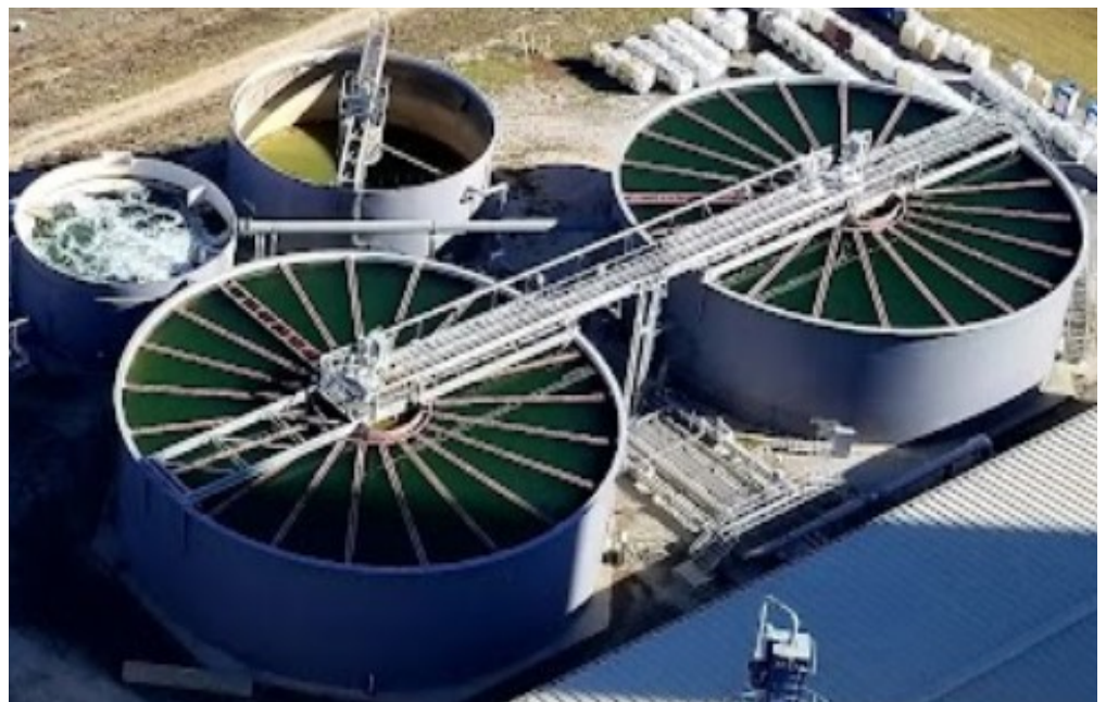
(2) 80' dia. Solids Contact Clarifiers and (1) 50' dia. Sludge Thickener
